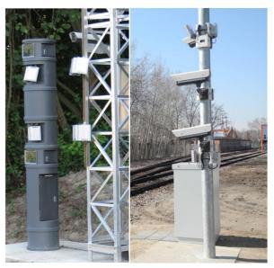
Optional add-ons for railway operators: Level detection for liquid or bulk materials, leakage detection or detection of open dome covers can be added at any time. In the event of an alarm, the unique assignment of the UIC number ensures clear identification of the corresponding wagon. Malfunctions can be solved immediately.
