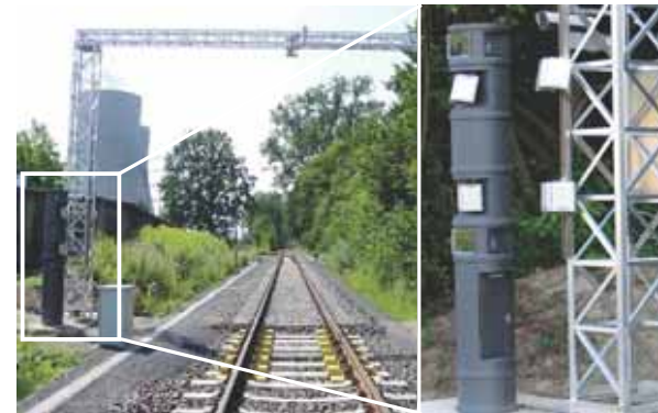
NUMBERCheck – Rail Gate.
